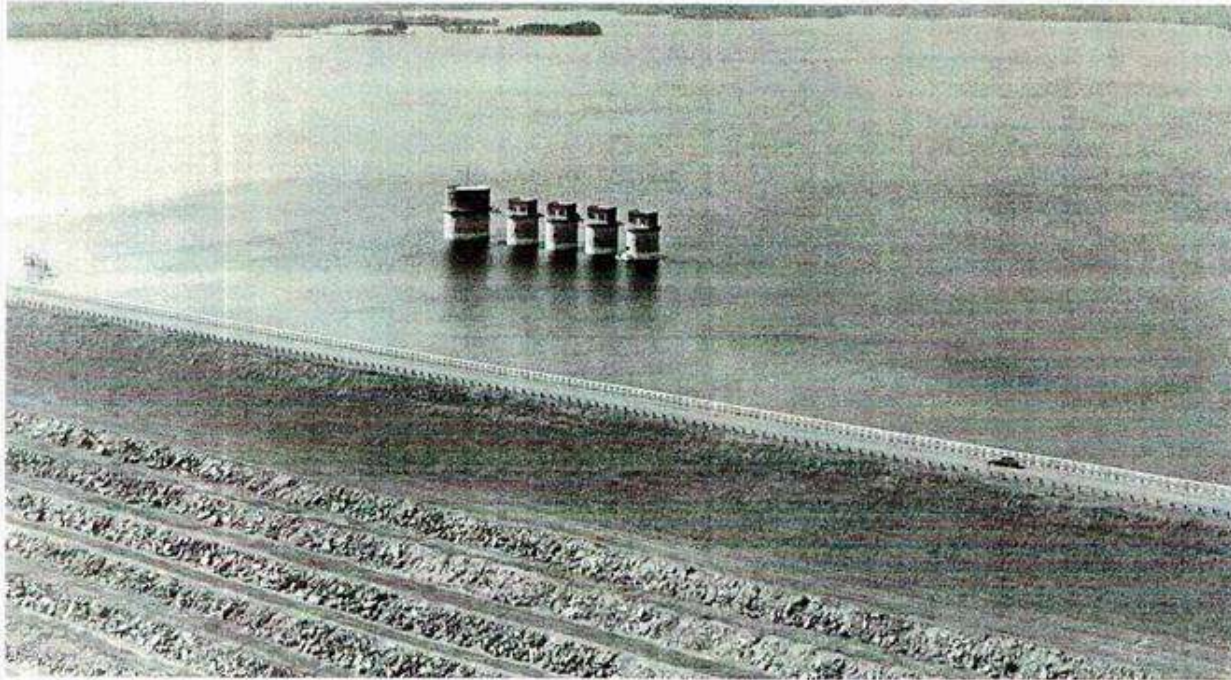
Water for boiler feed comes from 50,000-acre Lake Murray through these inlet pipes. The lake was created by the earthen dam seen in the foreground.
